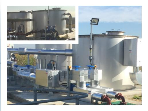
Work Carried Out: Insulate and clad exterior pipework.
