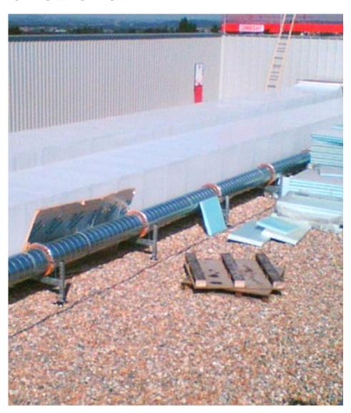
The roof top ductwork at the five story medical centre at Brierley Hill, Dudley was insulated by Rilmac Insulation with a brand new system called "Specialite".
