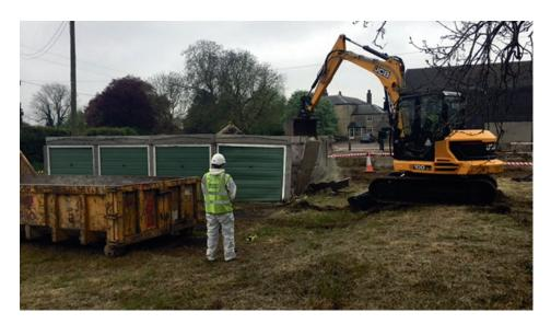
Rilmac were contracted to remove asbestos cement and demolish remaining structure of four dilapidated farm buildings and a garage block. Works involved hand removal of asbestos and machine demolition of the remaining structures. We had a specialist waste firm in to remove contaminated water. All works were completed in a 7 day programme by Rilmac employees. Project was completed on time and in budget.
