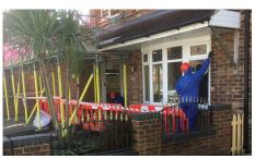
other volunteers could start work and the asbestos containing putty was removed from the window frames.
