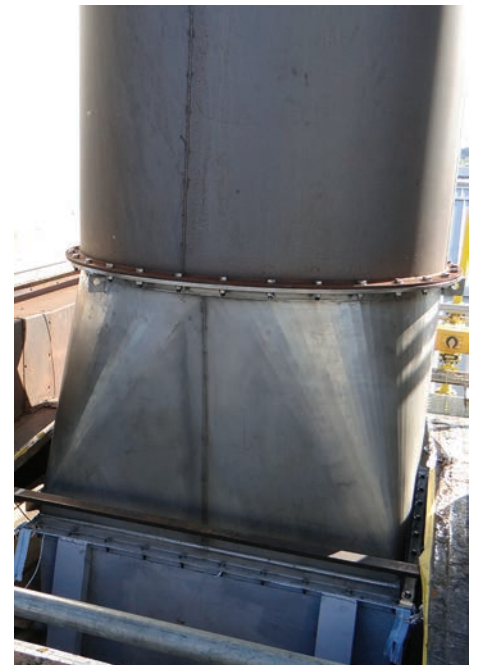
New ducting installed at SITL
