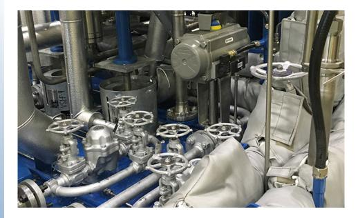
Installation of foil faced mineral wool insulation protected with stucco aluminium cladding to the Oil and Steam pipework on the turbine. Areas where it was not achievable to use previously stated methods such as valves and flanges, removable jackets were fitted and manufactured from a grey silicone cloth with a mineral wool insulation filling secured with Velcro and drawstrings.
